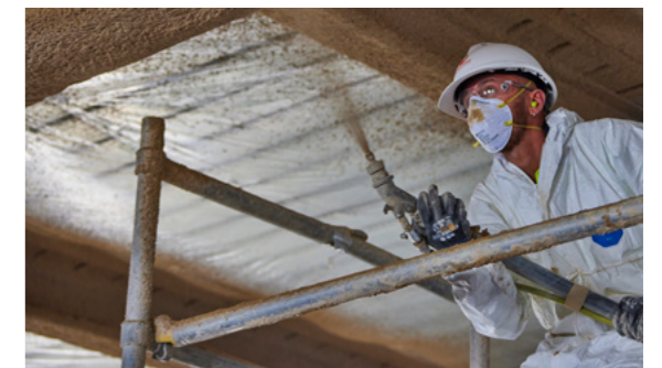
VERMICULITE FIRE SPRAY BEING APPLIED
