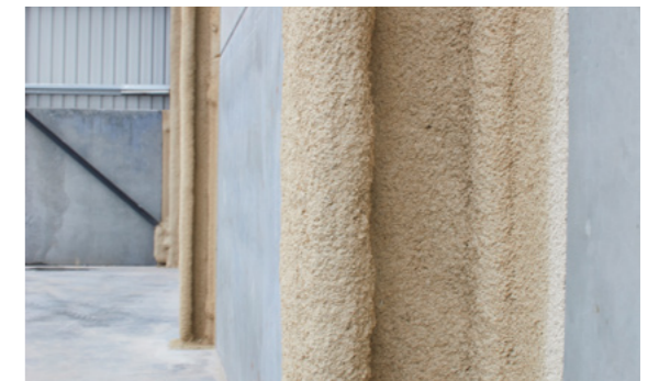
VERMICULITE FIRE SPRAY APPLICATION
