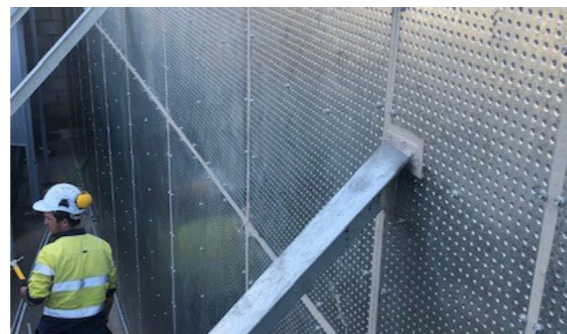
DURASTEEL® INSTALLATION, BILOELA
