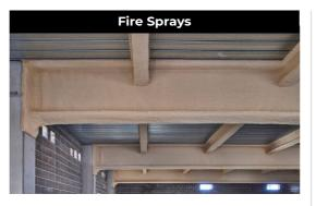
Wet mix Spray-applied Fire Resistive Material (SFRM) has been used in structural steel fire protection for decades. It is a low cost option and is generally used for internal environments as it is susceptible to damage by water ingress.
