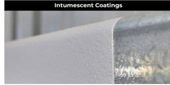
Intumescent is the newest fire protection methodology to come onto the market. Unlike boards and vermiculite, intumescent is a reactive material which expands to insulate structural steel in a fire event. Every intumescent has different material properties and therefore have different required thicknesses and expansion behaviour.
