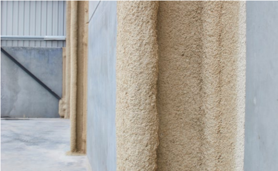
VERMICULITE FIRE SPRAY APPLICATION
