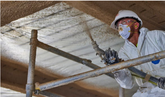
VERMICULITE FIRE SPRAY BEING APPLIED
