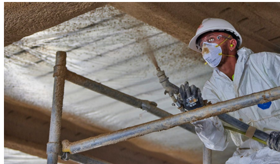
VERMICULITE FIRE SPRAY BEING APPLIED
