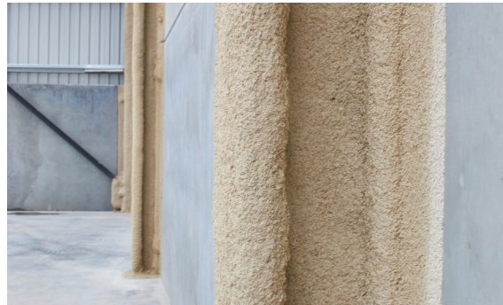
VERMICULITE FIRE SPRAY APPLICATION
