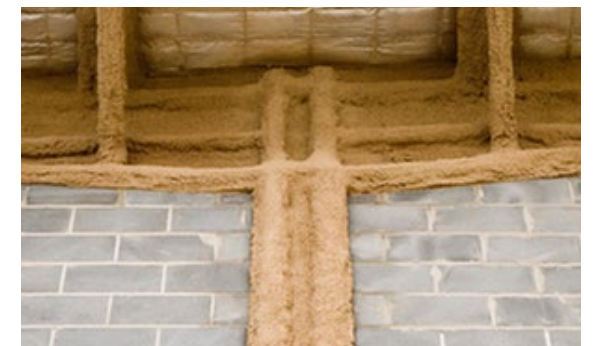
VERMICULITE FIRE SPRAY APPLICATION
