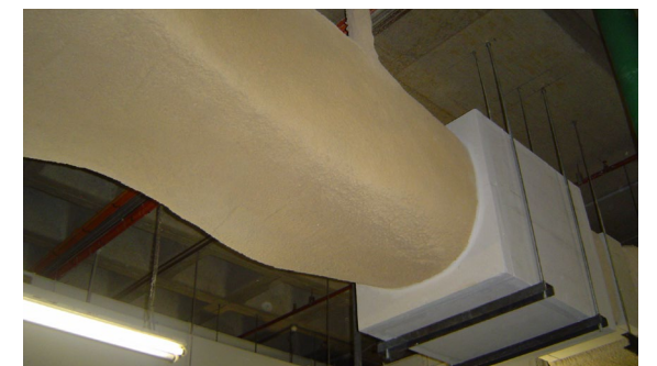
VERMICULITE FIRE SPRAY APPLICATION
