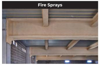
Wet mix Spray-applied Fire Resistive Material (SFRM) has been used in structural steel fire protection for decades. It is a low cost option and is generally used for internal environments as it is susceptible to damage by water ingress.
