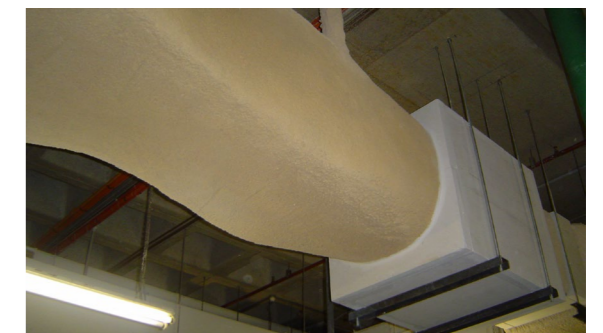
VERMICULITE FIRE SPRAY APPLICATION
